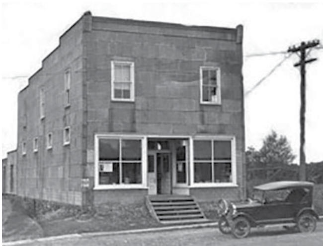
Wootten Maynooth General Store 1907, before the fire.
